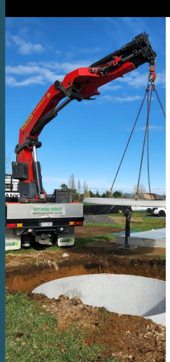
Our tanks are all delivered with a Hiab on the rear of our trucks. Each truck has a 53-ton crane positioned at the rear of the deck.
